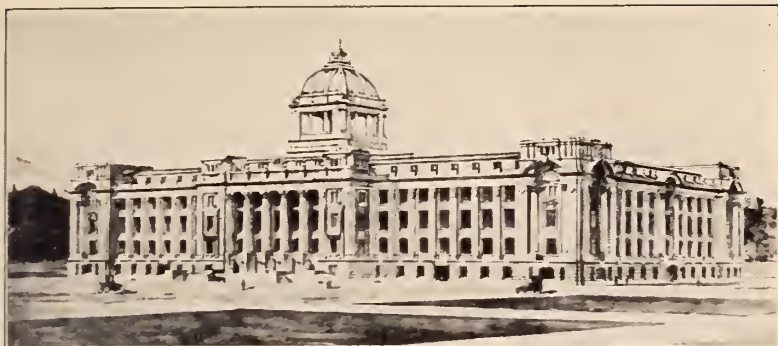
New Offices of the Government-General, Seoul. To be completed in 1924 at a cost of yen 3,000,000.
